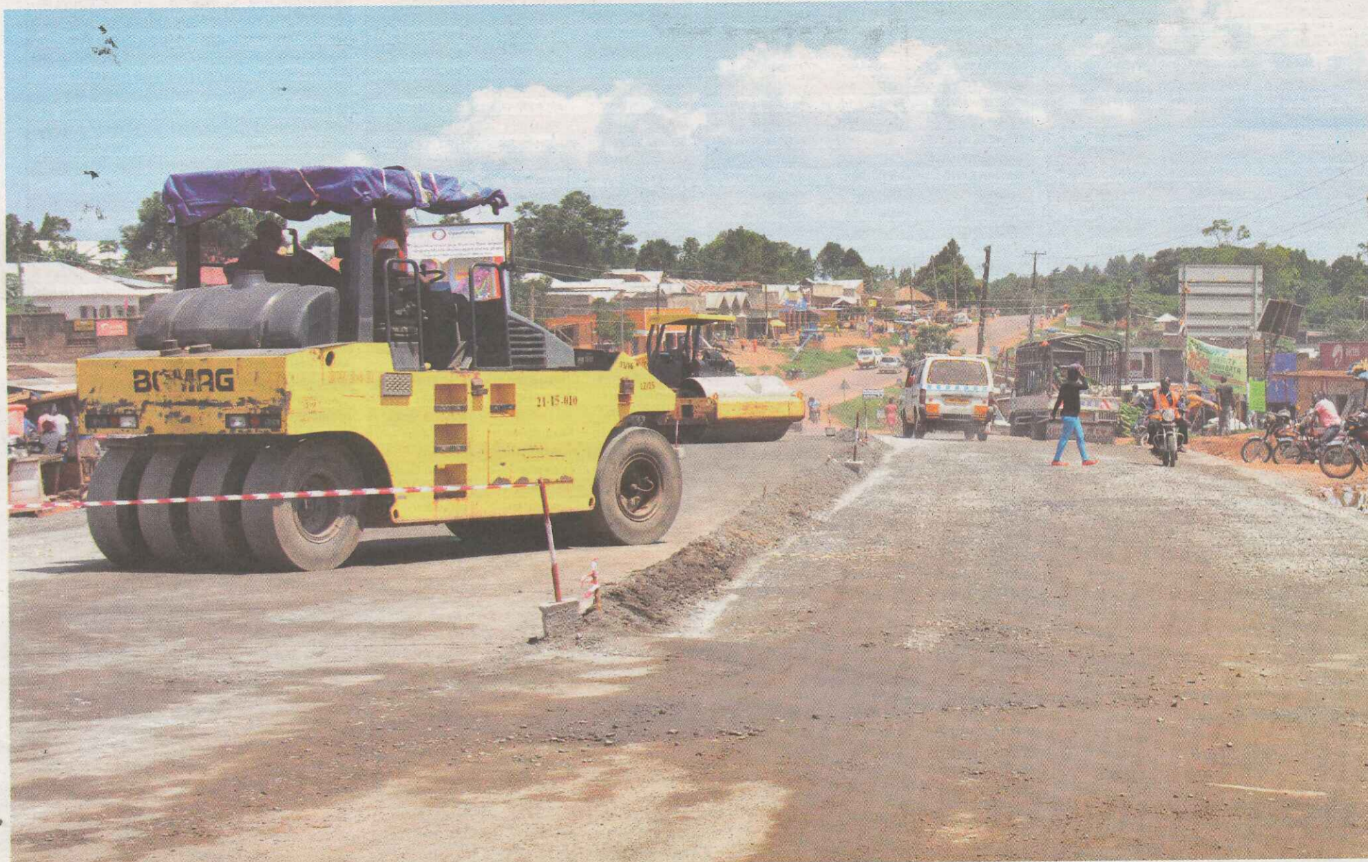
Construction. Earlier construction works on Kayunga road. COURTESY PHOTO
