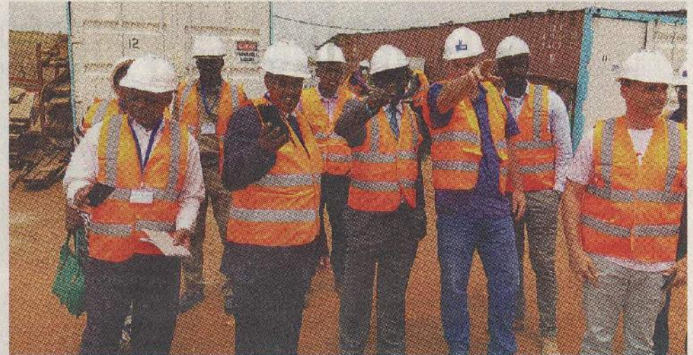
Isingoma and officials of KPCL and SBI Uganda touring the Kikagati Hydro Power Project site in Isingiro district recently. Photo by John Odyek
